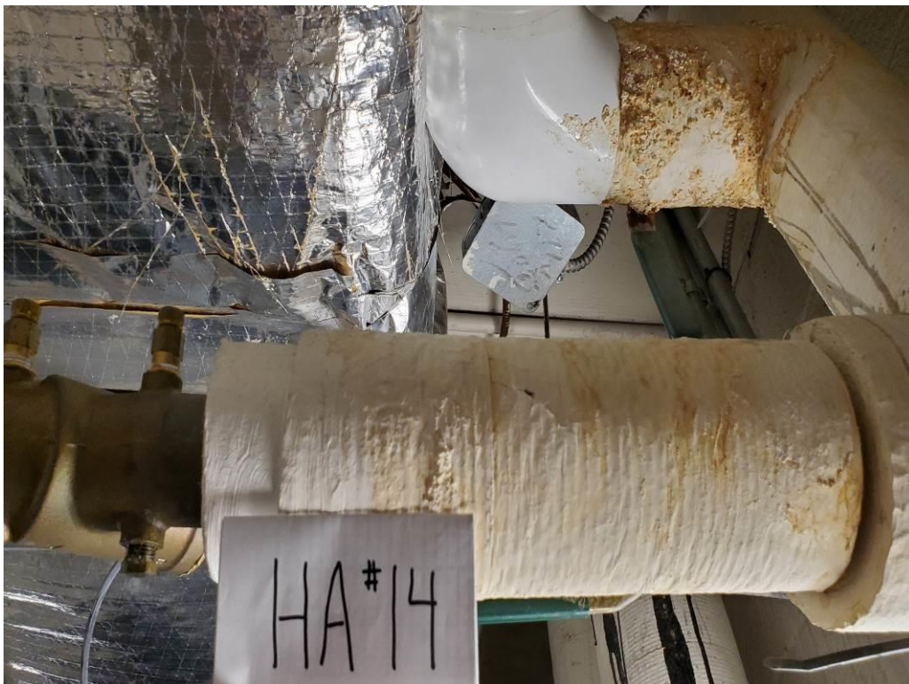
HA #14 – White Pipe Insulation Mastic
