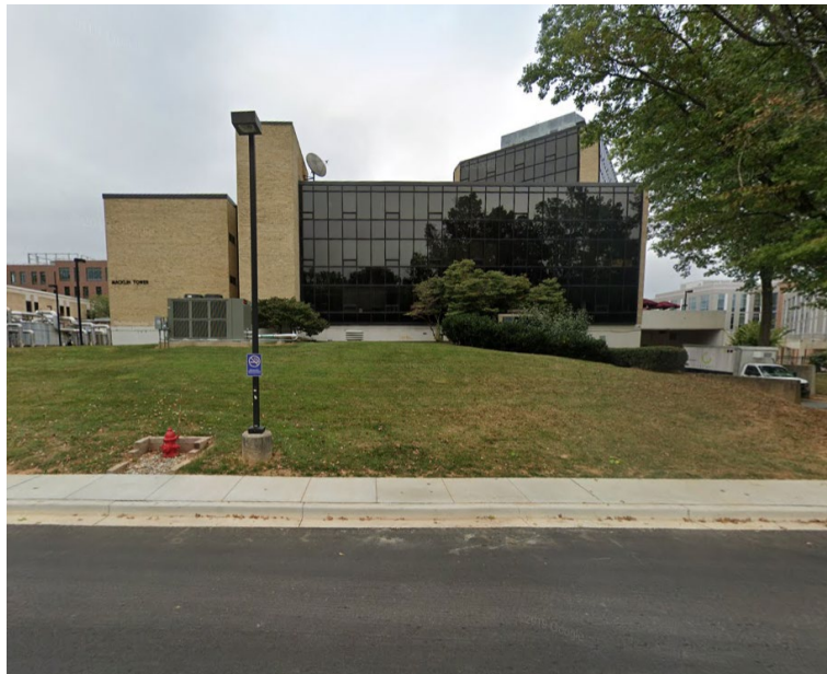
Figure 1-1 Photo of The Gordan and Marilyn Macklin Tower (Source: Google Maps)
