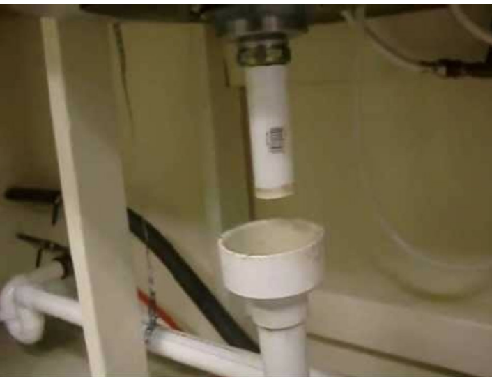
TYPICAL 2x3 WASTE RECEPTOR FOR HAND SINK
